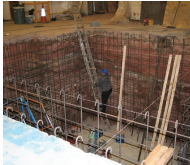
Work has already begun to make way for the new press
